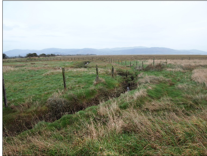
Plate 2.13: F1 Swamp – the main site drainage culvert discharges to an existing drainage channel to the north of the R172 Blackrock Road [December 2018]
